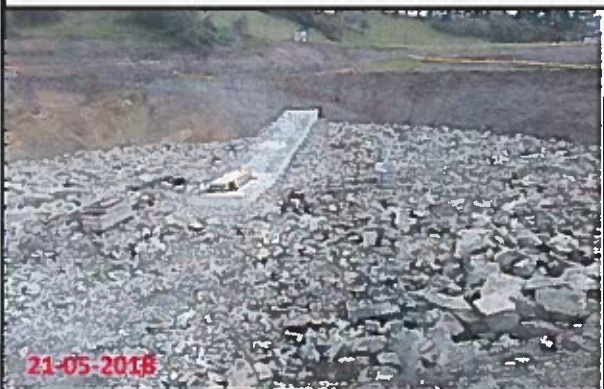
HORMIGON SIMPLE f'c = 140 \text{ Kg/cm}^2 PTAR019
